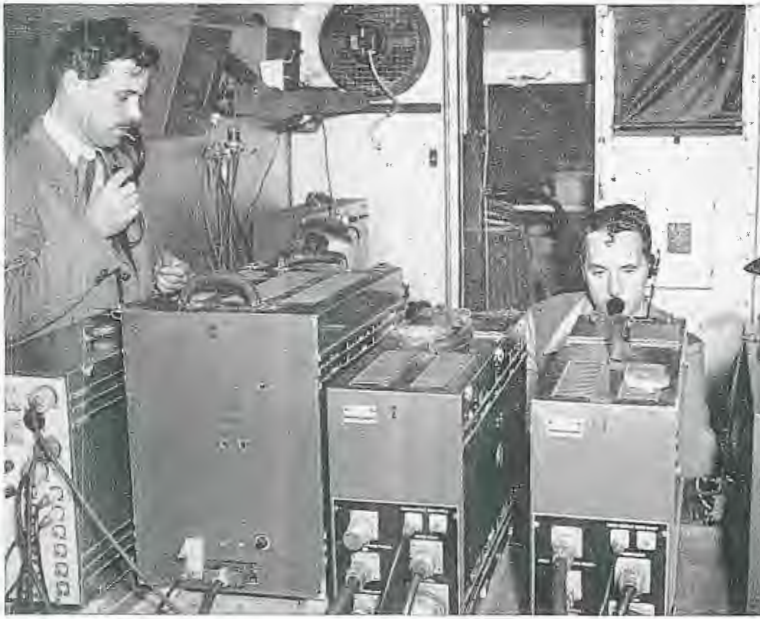
4. Cables from the cameras lead to the camera control units in the telemobile, interior of which is shown in this view.
