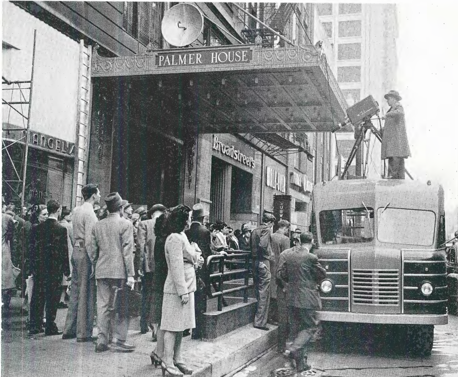
FIG. 2. The TJ-50A Mobile Unit on State Street, Chicago. Standard relay transmitter may be mounted on roof of unit or anywhere within 400 feet. In this view it is placed on hotel marquee for sending video signals to receiver at WBKB on State-Lake Building, three blocks north.
