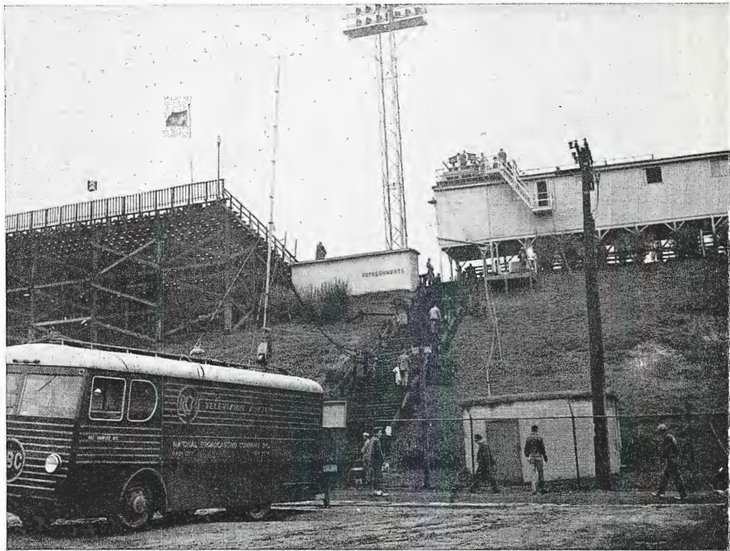
1. Overall view of the installation at Baltimore Stadium. The tele-mobile unit's old antenna mast served as a support for the camera, power, and microphone cables. The two cameras may be seen to the right of the lighting tower. The microwave transmitter and parabola is on a platform to the right of the top of the steps.
