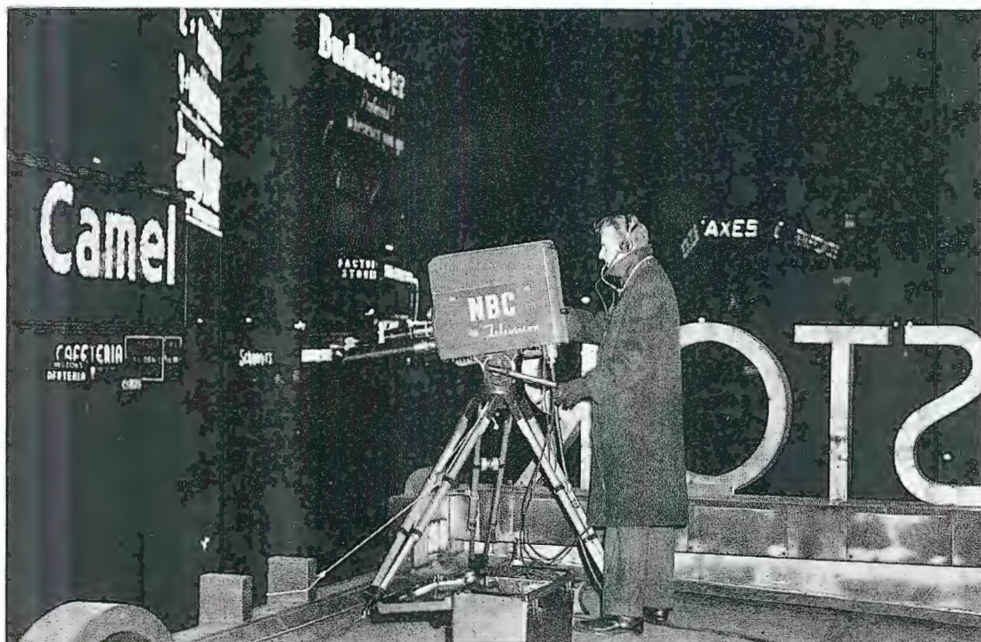
FIG. 9. Televising the New Year's celebration in Times Square from the Marquee of the Hotel Astor. Although the streets appear dark in the photo, the Image Orthicon successfully picked up the crowds.
