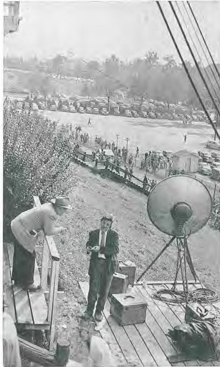
5. From the control position video signals were fed to the microwave transmitting equipment which was mounted on a specially-built platform, as shown here. This photo was made prior to the r-f test, during the equipment setup.
