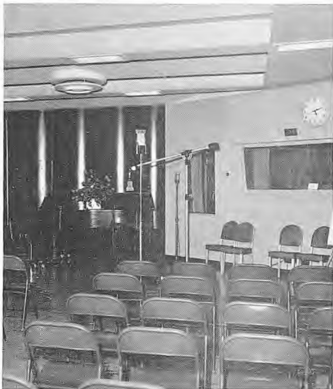
FIG. 1. Front view of main studio (note polycylindrical surfaces on wall and ceiling).
